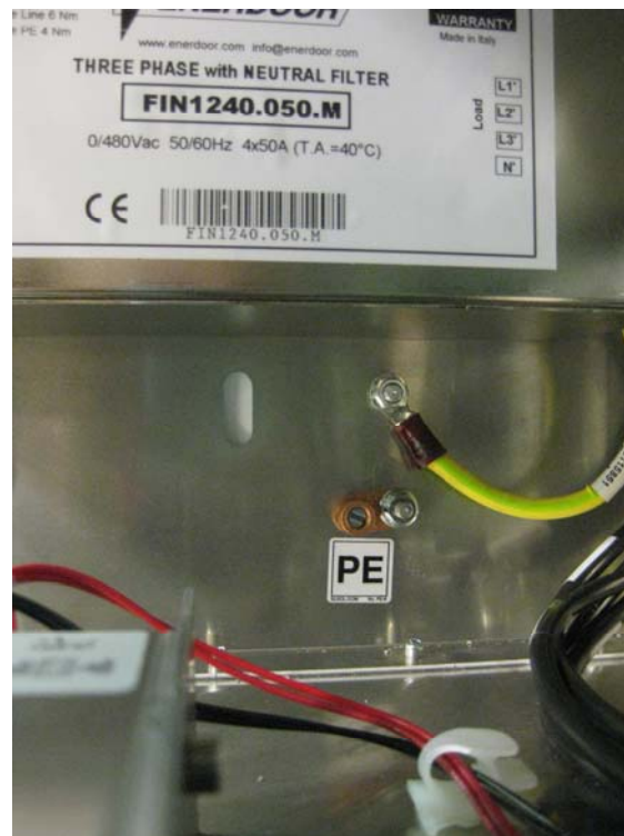
Figure 9 – PE Terminal located on the inside of the E-Box.
